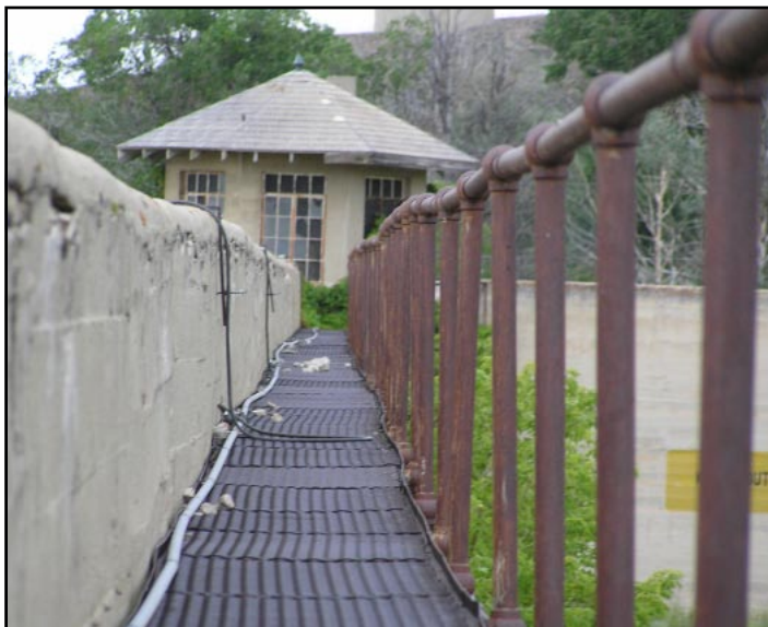
The existing concrete walls and associated towers were built following a mass escape of 28 inmates in 1912.
